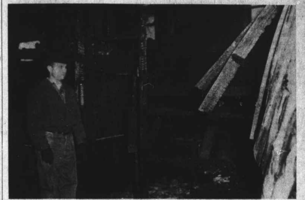
FIRE STARTED HERE.—Gale Scroggs, manager of Watauga FCX, stands near where it is believed Friday night fire in the store started. Offices behind Mr. Scroggs were also damaged.—Staff photo.
