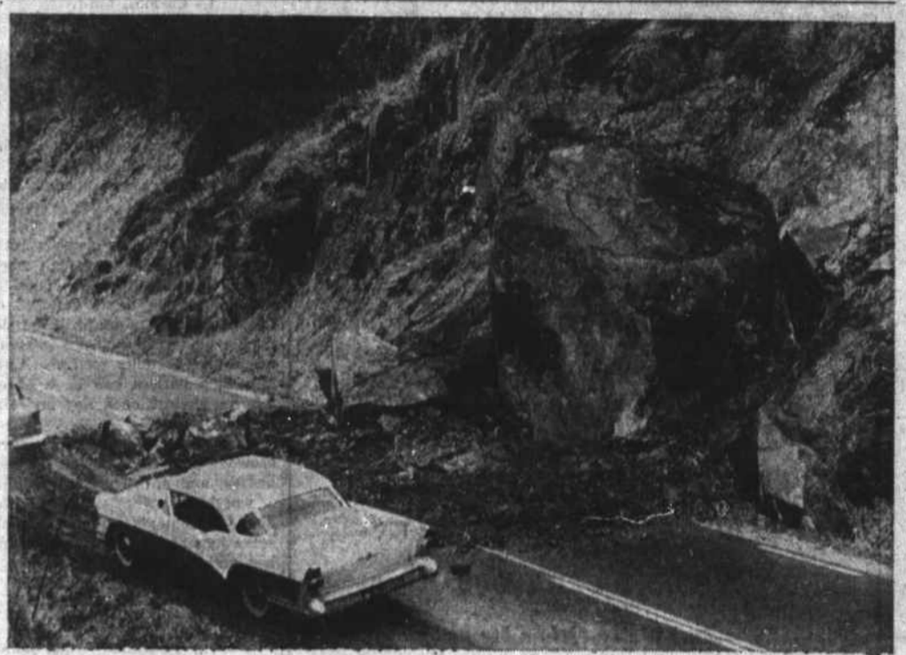
ROADBLOCK —The week end rain caused huge rock (near right) to slide from the mountainside Saturday morning, and send tons of smaller rocks and earth across U. S. 321, near Boone Golf Course entrance. One-way traffic was being maintained at the time George Flowers made this picture. Highway crews cleared the way and normal traffic was resumed later in the day. The rock was said to have measured more than twenty feet across.
