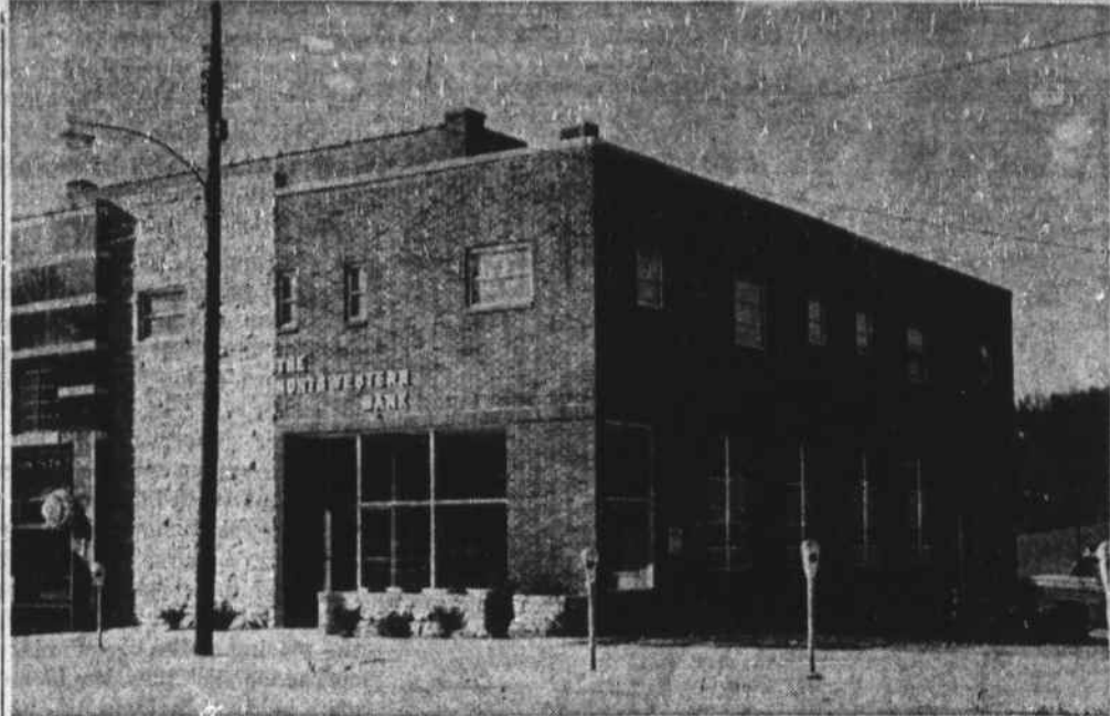
OPENS MONDAY —The above offices of the Boone branch of The Northwestern Bank will open for business Monday morning. The building, started last fall, has just been completed, and is said by bank officers to be the most modern structure of its kind serving Northwestern North Carolina.
