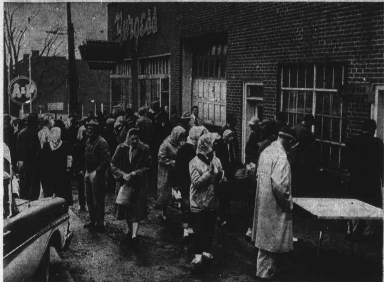
FIRE SALE. —These people were waiting Saturday morning to get in to the fire sale at Burgess Furniture Store. Shortly before this picture was taken, someone estimated that more than 300 people were on the outside waiting for the store to open. Although it rained most of Saturday, business was brisk in town, and traffic was almost at a standstill at times on the Street.
