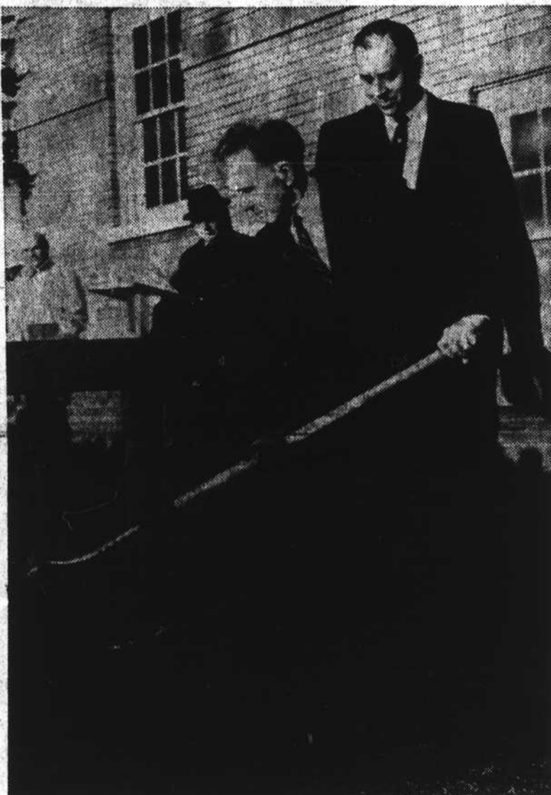
Mr. A. L. Cook turns first shovel of dirt at the ground-breaking ceremonies which started the huge expansion program of the First Baptist Church.—Flowers photos.
