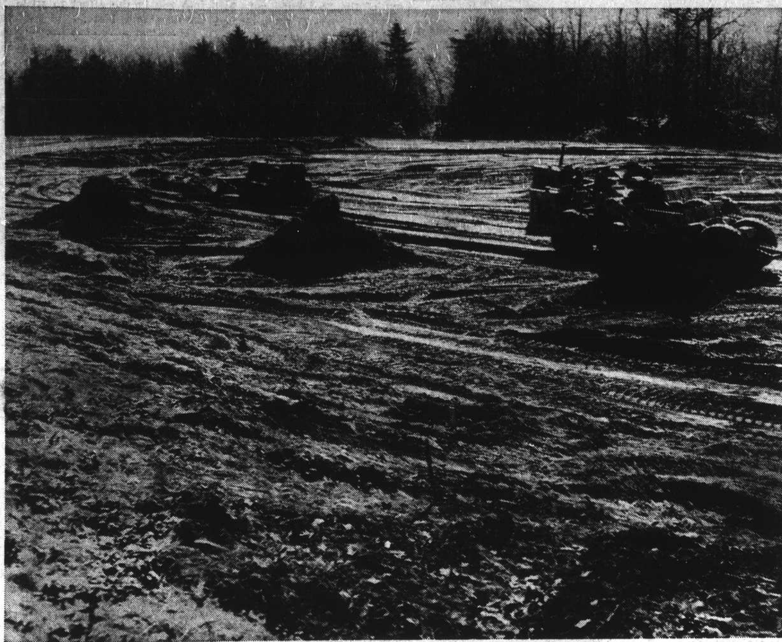
GRADING ALMOST COMPLETED AT NEW PLANT SITE. (Minor photo.)
