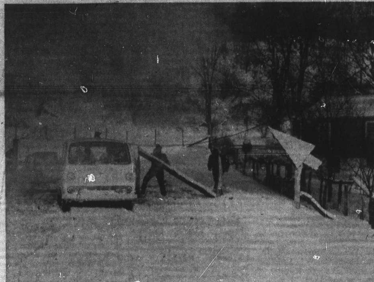
A HIGH-VOLTAGE WIRE FELL ACROSS A TRUCK adjacent to the burning Fox Brothers Grocery, when firemen were rescuing a car which was parked behind the building. The fireman was warned to stay inside, since the wheels of the truck acted as conductors. Another fireman was nearly hit by the wire which fell off the back of the truck as it pulled the car forward. (Rivers photos.)
