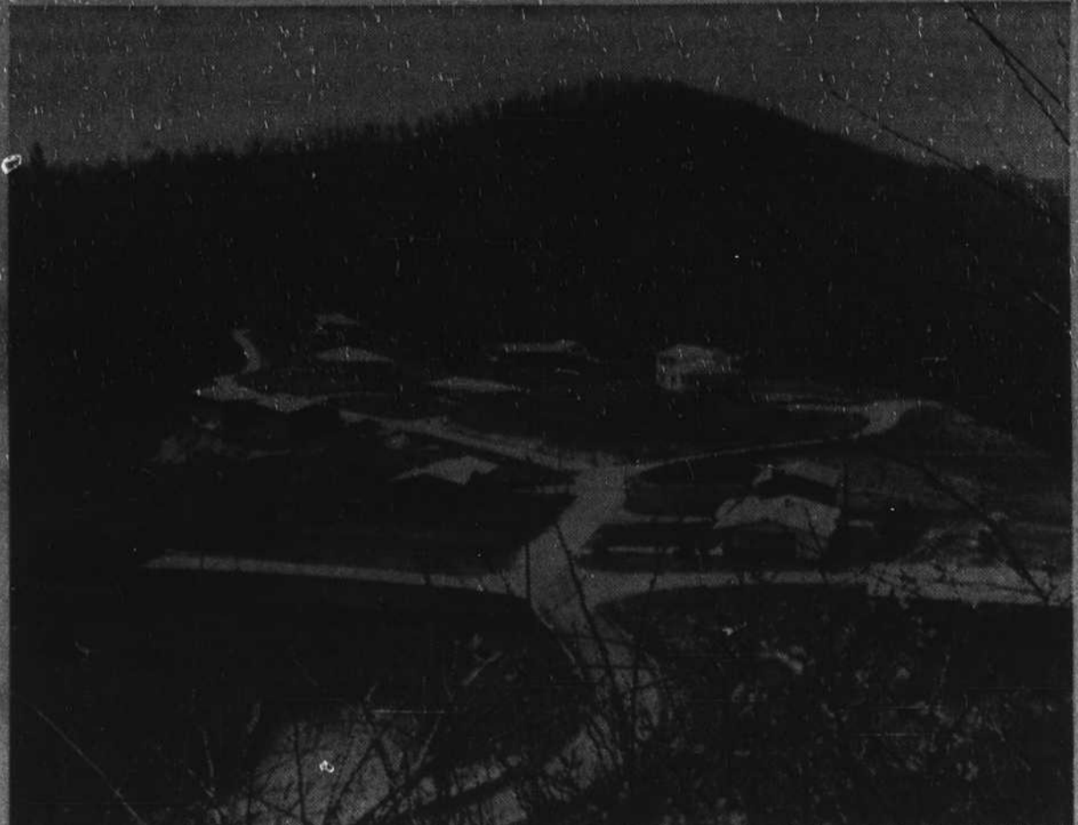
HERE ARE A FEW OF THE 17 HOUSES constructed at the summit of the Poplar Hill housing development after Patrolman William D. Teem built there five years ago. As rapid as the summit growth has been, it probably does not comprise a fifth of the number of houses which have sprung up along Poplar Hill Drive and adjacent property. (Rivers photo).
