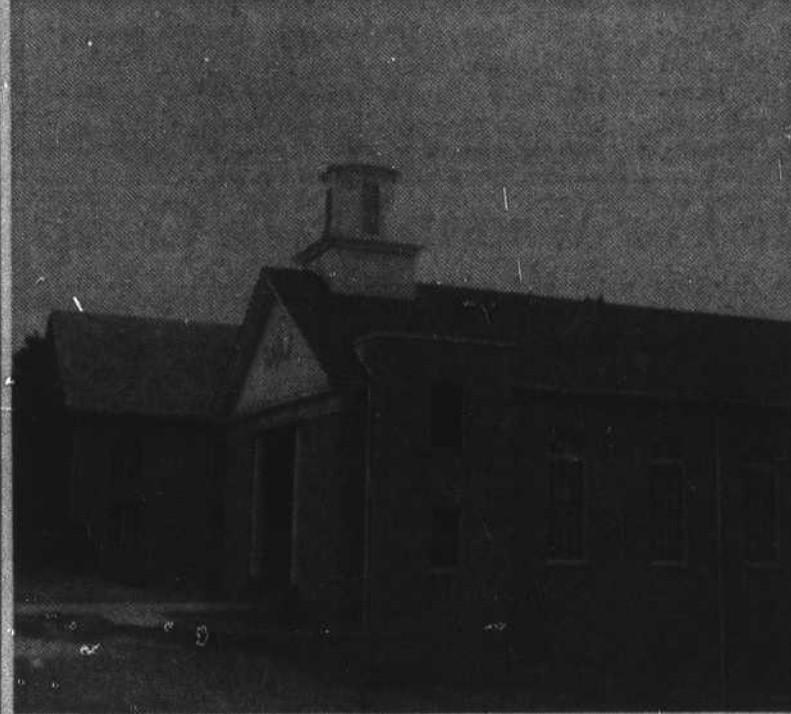
NEW ADDITION TO CHURCH PLANT.
