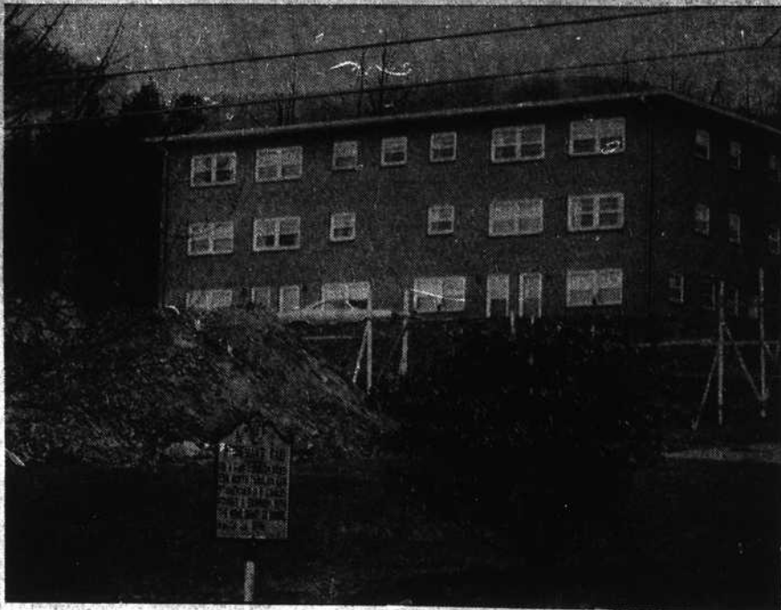
AN 18-UNIT EXTENSION is being built onto the Queen Street Apartments, seen here from West King Street. Stanley Harris Sr. says he has sold the apartment building to a Fayetteville, N. C., group, who purchased the Phillips property, adjacent to the County Court House, for the expansion. (Staff photo)
