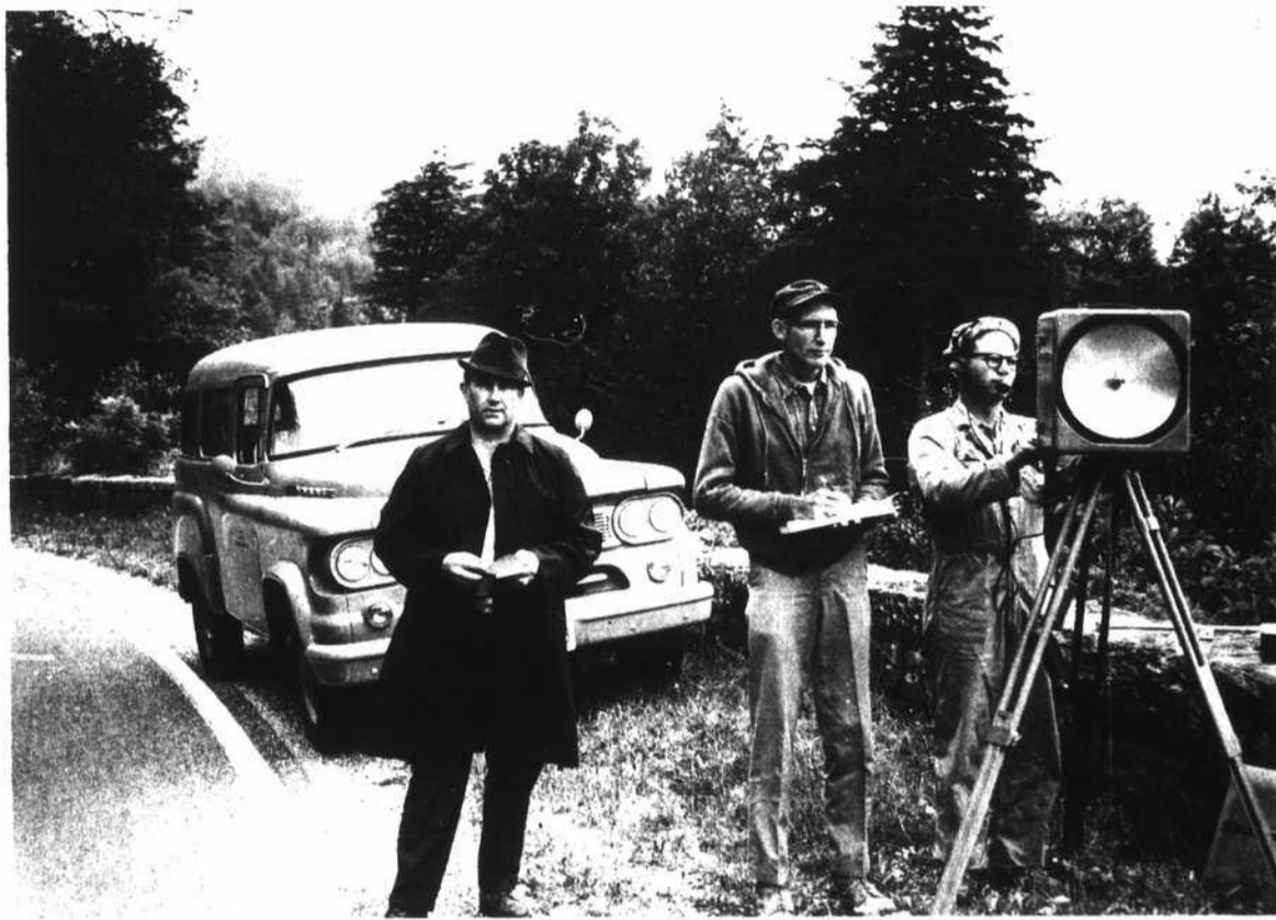
WORK ON PARKWAY LOCATION —J. R. Jenson, left, Regional Locating Engineer, Bureau of Public Roads headquarters, Arlington, Va., has started work on the last part of the Blue Ridge
