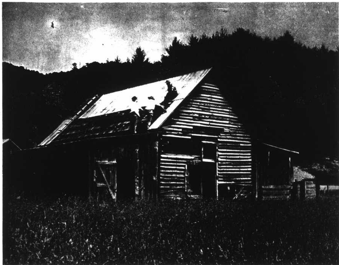
PLANNED MOVE OF SCHOOLHOUSE —The old Shulls Mills School is shown as it stood four years ago before being moved to the Horn in the West grounds. Shown planning the moving task are (l-r) Bob Allen, director of Public Affairs, ASTC;
