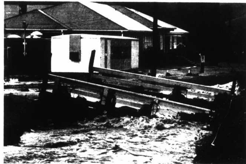
STATE BRIDGE OUT—District Highway Engineer Tom Winkler estimates the loss of the state bridge from old Highway 421 to Mabel School between $6,000 and $7,000. The bridge must be replaced, he said, because of the severe damage done to it in Thursday's flash flood.
