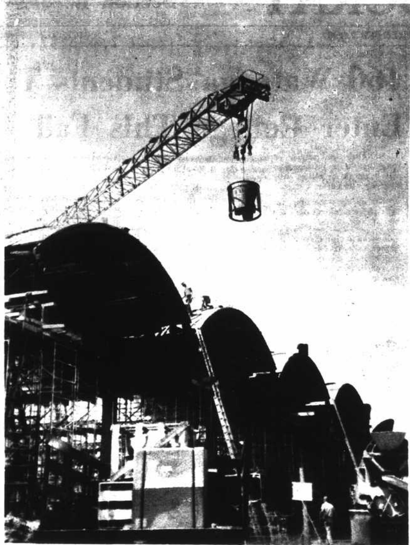
THESE "HUMPS" OF STEEL are an architectural feature of the gym being built at Appalachian State University and dramatize the ultra-modern aspects of the construction. All concrete and cable beaming has been poured. (Staff photo)
