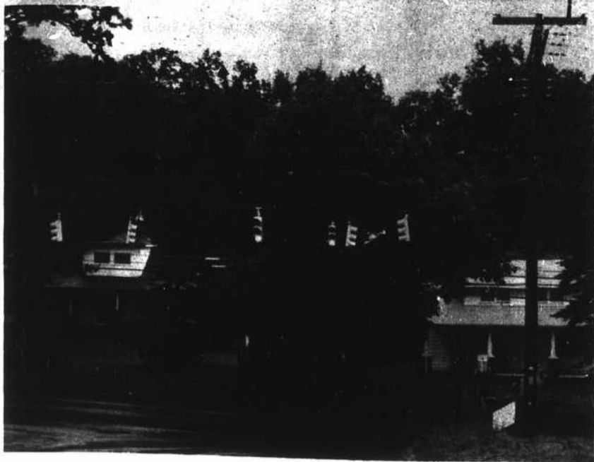
THE CITY has installed traffic signals at the intersection of East King Street and the Highway 105 Extension. The work was done under the supervision of the Highway Department.
