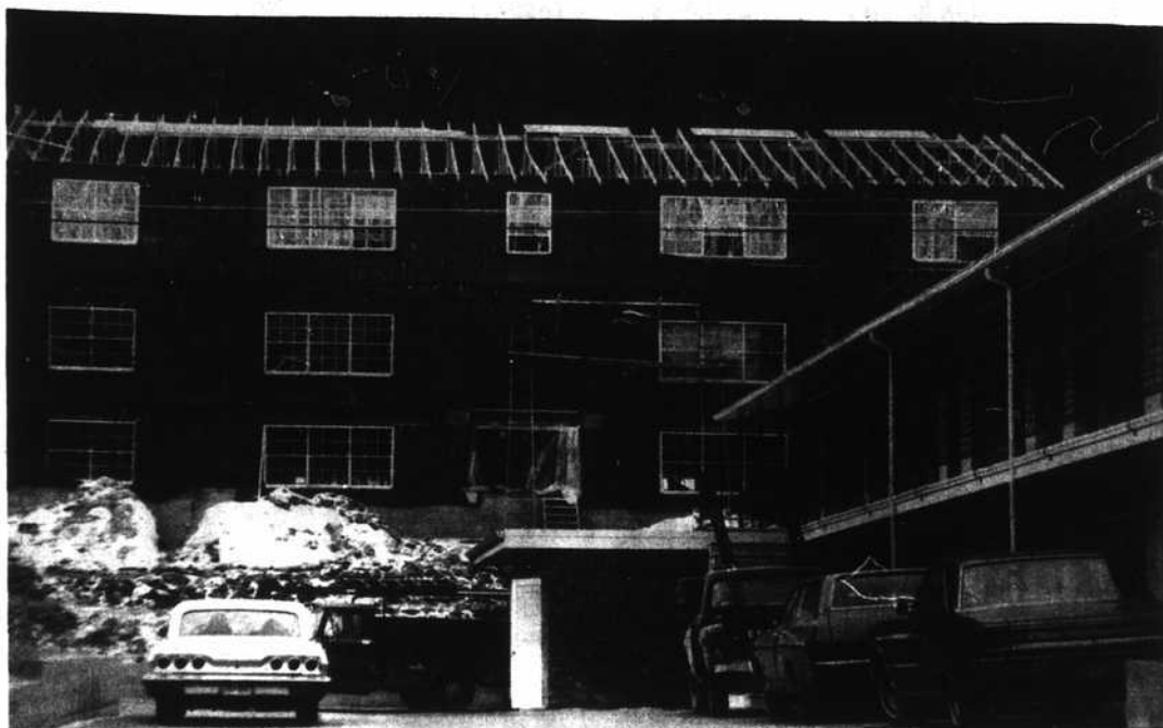
220 UNITS GOING UP—With an obvious endorsement for the growth of the town and Watauga County, Larry Maher of Boone is putting up a huge apartment complex adjacent to Appalachian
