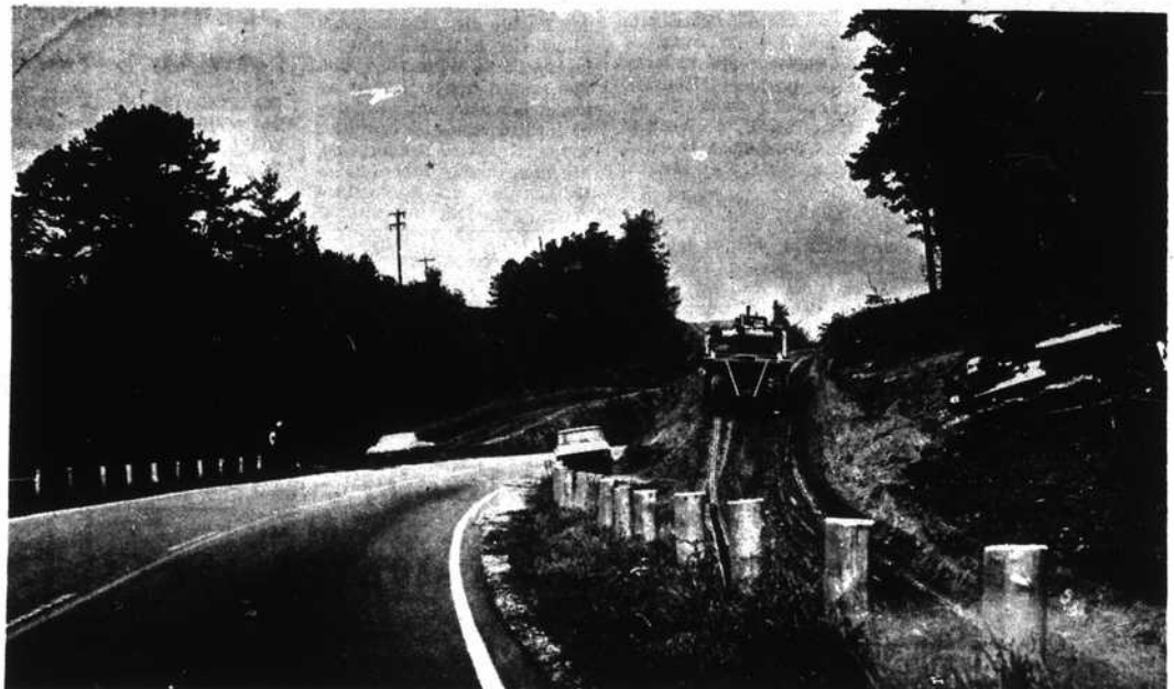
FASTER TRAVEL UP THE HILL—Soon the passing zones will be able to pass the heavy trucks, greatly facilitating the mountain to Blowing Rock will be completed. Then motorists travel to the noted resort.—Lenoir News-Topic photo.
