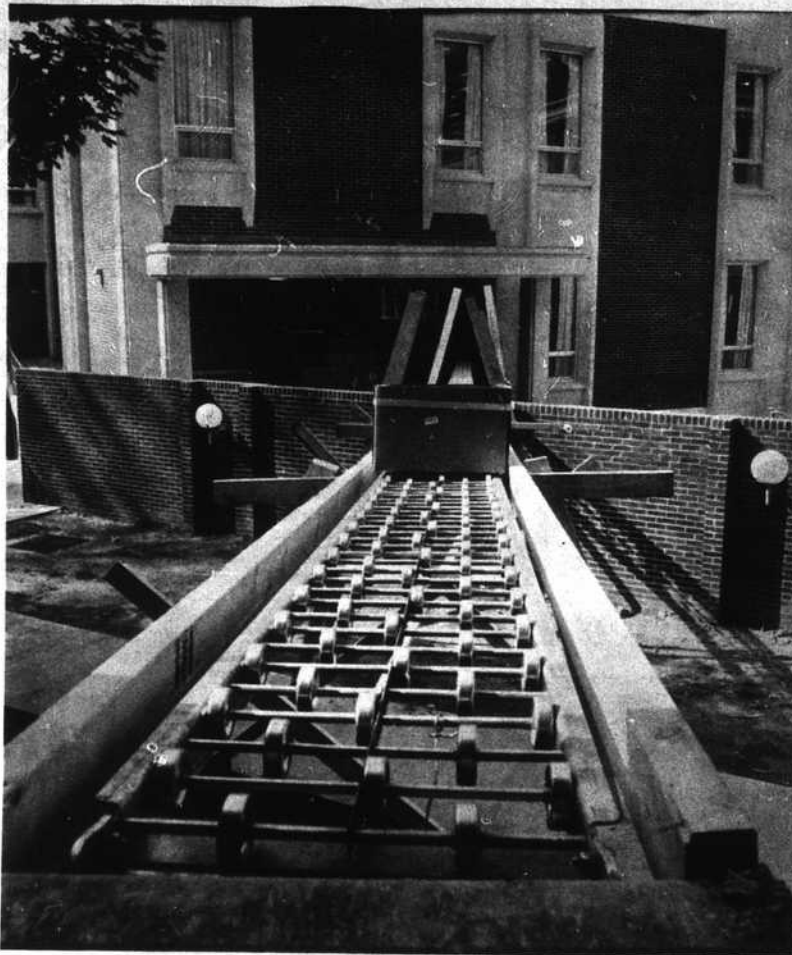
ROLLERS TRANSFER BOOKS—Scaffolds supporting lengths of steel rollers are making the task of transferring the rash of books from Appalachian's old library building to the adjacent new library. Heavy boxes filled with the volumes are being sent down the inclines to various rooms in the structure with scant time needed for the transfer. In the top picture, a large box rolls downward toward the inside of the recently-completed building.
