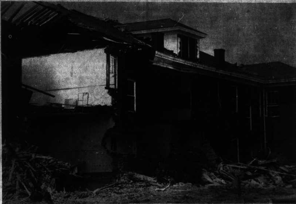
LANDMARK GOES—The old elementary school building, long familiar to the Appalachian University scene, is being swept from the campus by wrecking crews. The building, whose doors were first swung open to Boone area students in 1925, housed the ASU student book store just prior to its demolition. It
