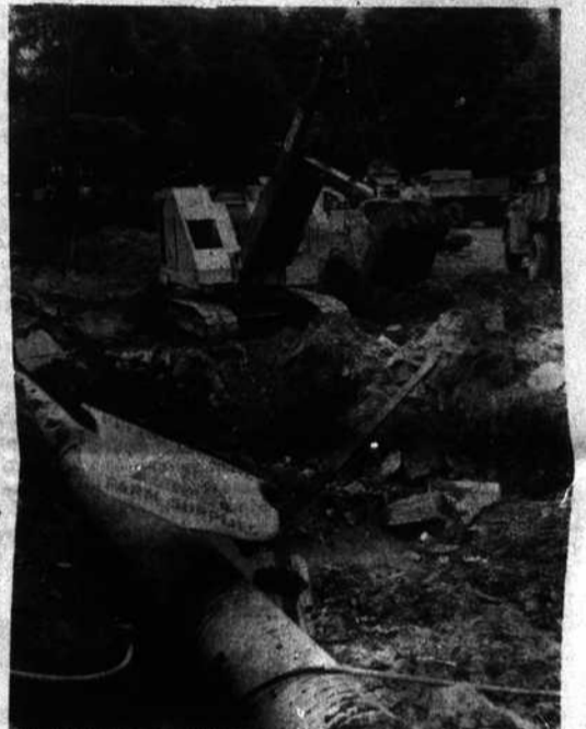
ROAD CLOSED—The Highway Department shut down travel on South Water Street beginning early last week to replace what District Engineer Tom Winkler termed "an undersized culvert." Five or six years ago, he explained, the bridge across Boone Creek was taken out and replaced with the pipe. Since then the manager of the FCX Service next to the creek complained the inadequate pipe had backed water into his building causing damage to a motor during one freshet. The FCX asked for a drainage survey and when the Hydrographic Department in Raleigh investigated, Winkler said they agreed. (Staff photo)
