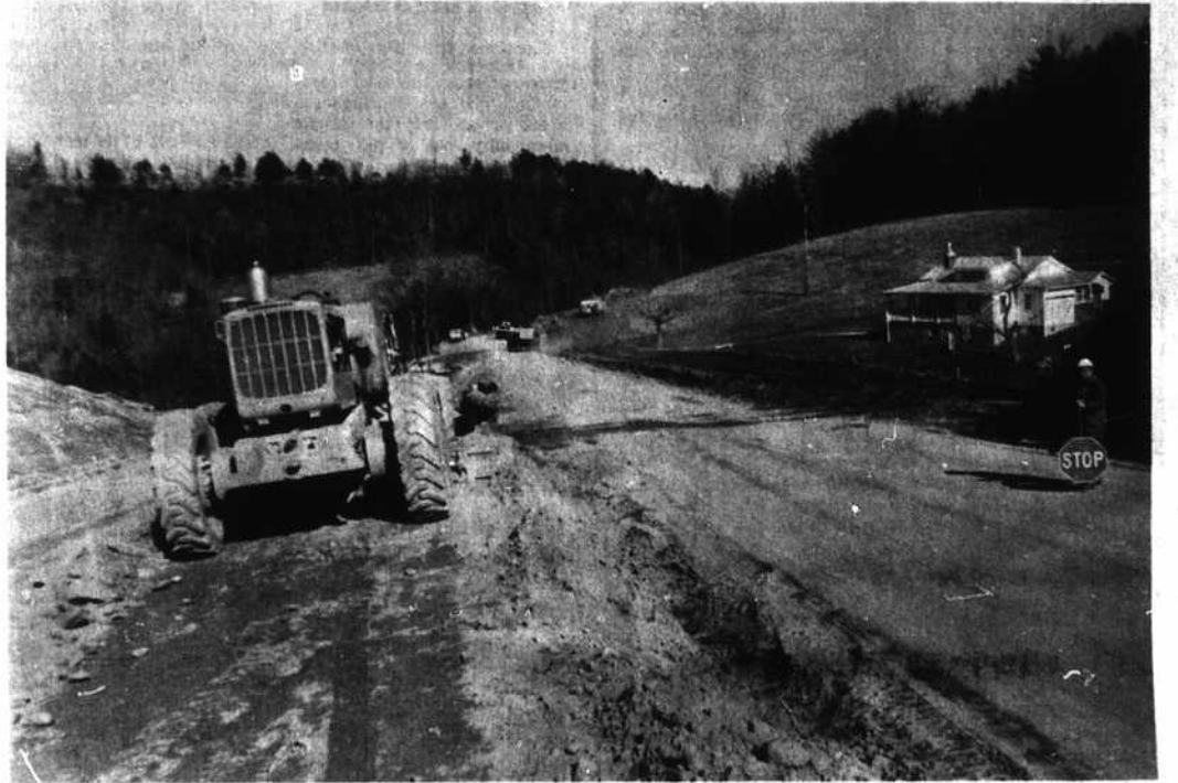
TRAFFIC IS BEING MAINTAINED DURING CONSTRUCTION
