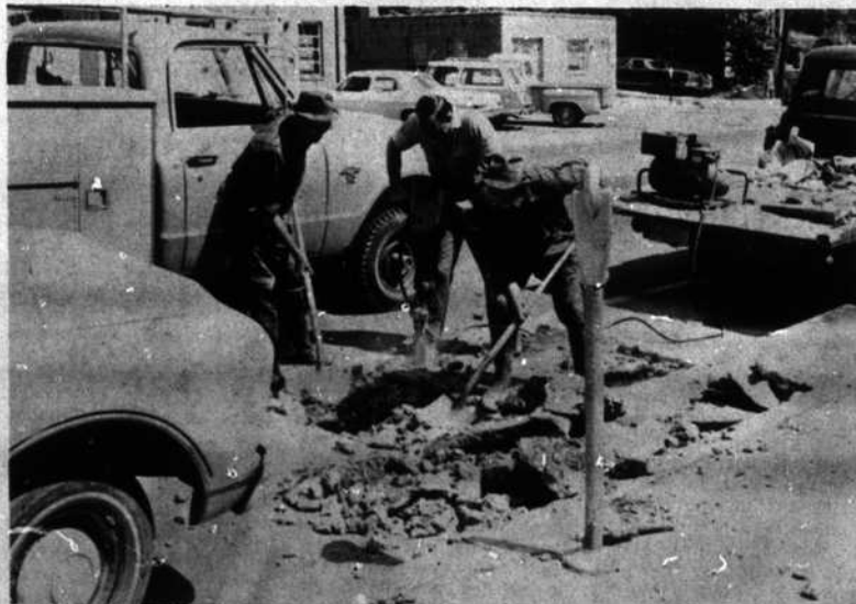
City workers Roby Greene, Benny Greene and W. W. Austin break up the pavement on West King Street during an assignment to connect the water line from the Bill Hodges building to another line. The line formerly used had rusted through. The city used pressurized water to flush a route for the new connection under West King Street instead of having to tear up the asphalt. (Staff photo)
