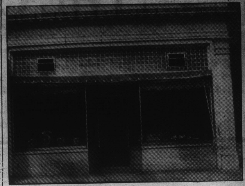
Since 1934 Campen's, Edenton's modern jewelry store, has occupied this attractive up-to-date building located adjacent to the Taylor Theatre.
