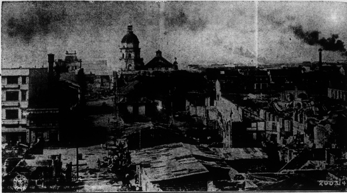
MANILA CITY IN FLAMES—Fires destroyed a large part of the downtown section of the capital of the Philippines upon the approach of the American troops. During the night TNT, planted by the Japs, exploded. Buildings were wrecked and fire added to the devastation.
