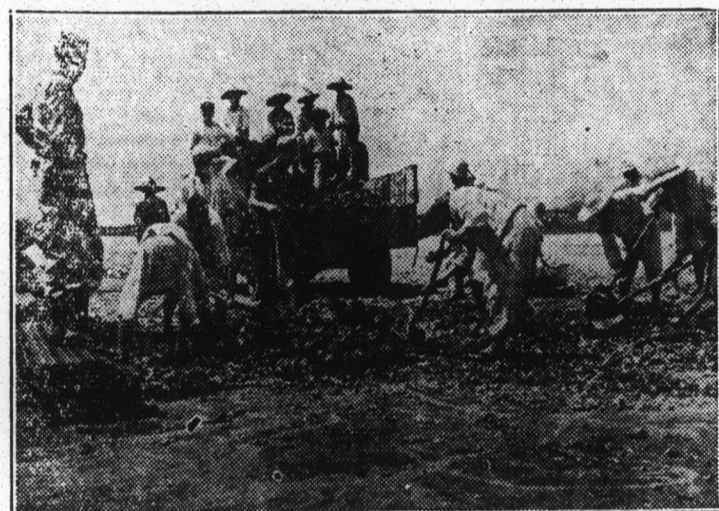
AVIATION ENGINEERS WORK KOREAN STYLE—Before adequate modern equipment was available, a small detachment of U. S. Army Aviation Engineers supervised Korean laborers in repairing this damaged runway. Supplies for the ground forces in the front lines were airlifted to this strip and then sent to their destination by truck and rail. Standing in the left foreground is Captain William Turner, in charge of the Engineers in this South Korean
