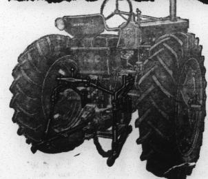
HERE'S "pick-up-and-go" farming at its modern best-the John Deere No. 800 Three-Point Hitch, which brings small-tractor convenience and utility to owners of powerful John Deere "50," "60," and "70" Tractors.
