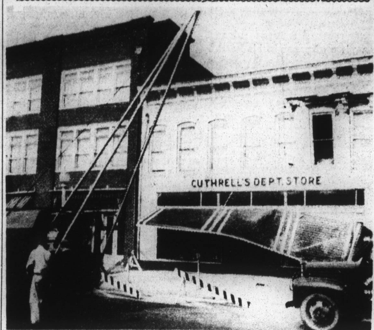
Above is seen the boom on an Electric and Water Department truck which hit a wire extending across Broad Street from Cuthrell's Department Store to the Hughes-Parker Hardware Store Tuesday morning of last week. The wire was used for Christmas decorations and pulled out a portion of the Cuthrell building and falling bricks ruined a metal awning. Nobody was hurt in the accident and damage was estimated at several thousand dollars. —(Evelyn Leary Photo.)
