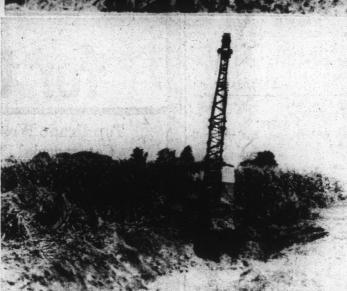
Some idea of improvement in drainage in Chowan County through civil defense funds is reflected in the above two pictures. In top picture is a view of a drag line at work in the Tiptoe Swamp, while the bottom photo shows a drag line at work clearing out and widening the Liza's Bottom ditch from E. L. Ward's pond to a point beyond Albemarle Street which carries off a large portion of Edenton's drainage water.
