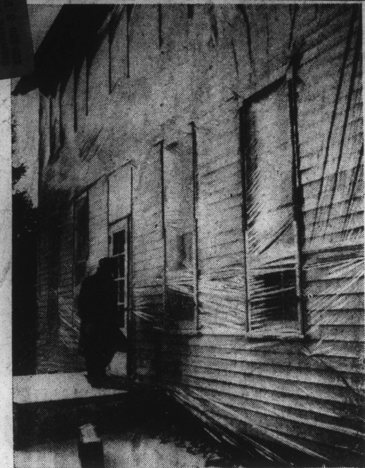
WRAPPED FOR WINTER —Wrapped in shimmering polyethylene, this old house in Lafayette, Ind., is the result of one cold winter night when the temperature fell to 10 degrees below zero. The goldfish bowl in the living room froze over, despite the fact that the oil burner was on. Purdue University Agricultural Experiment Station suggested wrapping the poorly insulated building in polyethylene film. Agricultural engineers are still testing the temperatures inside and out, but the residents of the house have been able to turn down the oil burner at night, even in coldest weather.
