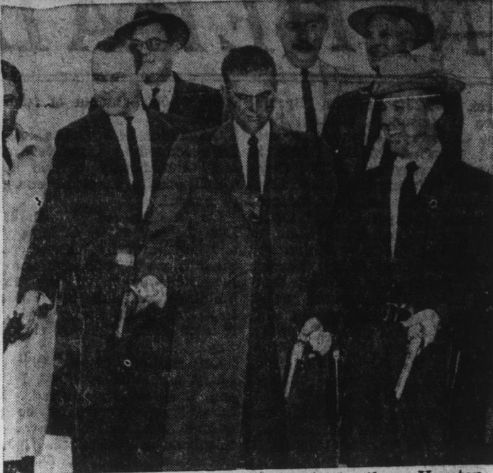
WHAT'S DOIN'—Totin' authentic pistols, these Houston Colt 45s National League baseball club officials hold a unique ground-breaking ceremony. They pump the ground full of lead to officially launch construction on a stadium.
