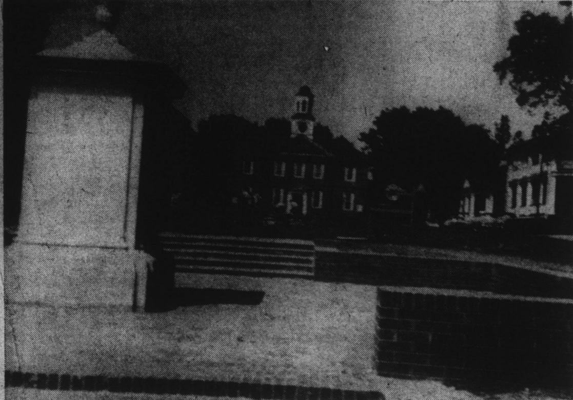
Pictured above is a view of the Joseph Hewes monument on the Court House Green, around which a plaza has just been completed by the Edenton Woman's Club. In front of the monument a neat brick sidewalk has been constructed and brick steps are on the green, as well as at the entrance to the Green in front of the Court House on King Street.
