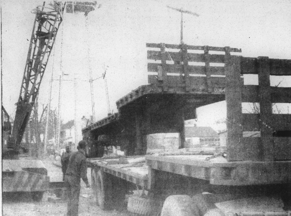
PIGGYBACK —Last week two flat bed trucks delivered four giant transformers to the Electric & Water Department on Freemason Street. One truck arrived Tuesday, the other Thursday. The driver of the first truck unhitched and returned to his home base, leaving the trailer to be returned by the second truck, arriving Thursday. Once the cargo was unloaded, Waff Brothers used their crane to pick up the trailer and place it on the other. Here you see the operation where a trailer goes for a ride—piggyback.
