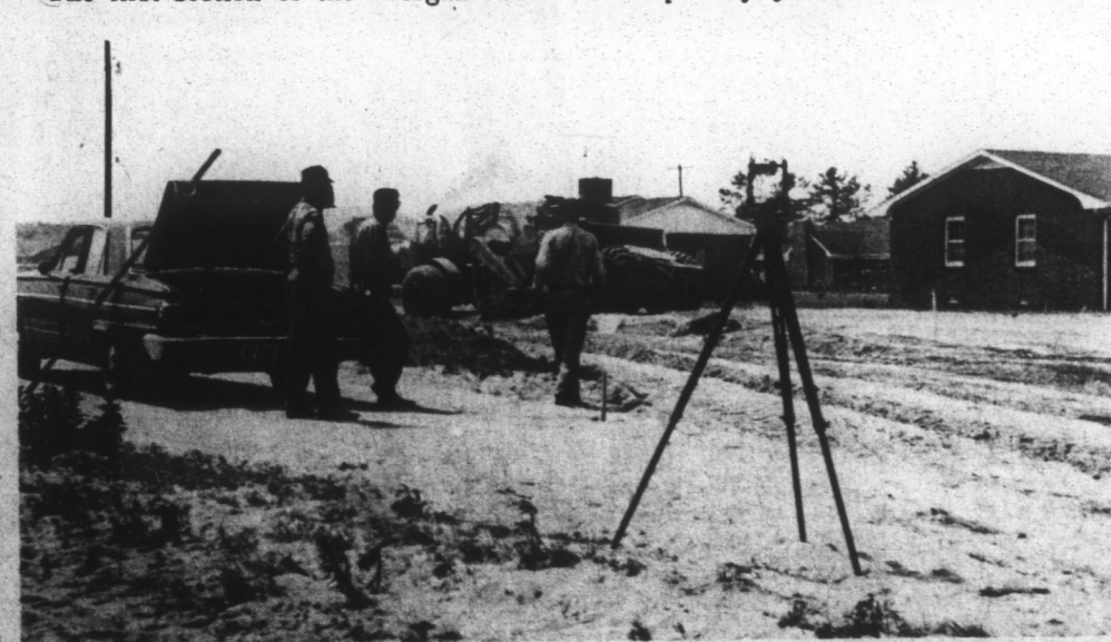
Jones Studio Photo Work Underway on New Section of Morgan Park
