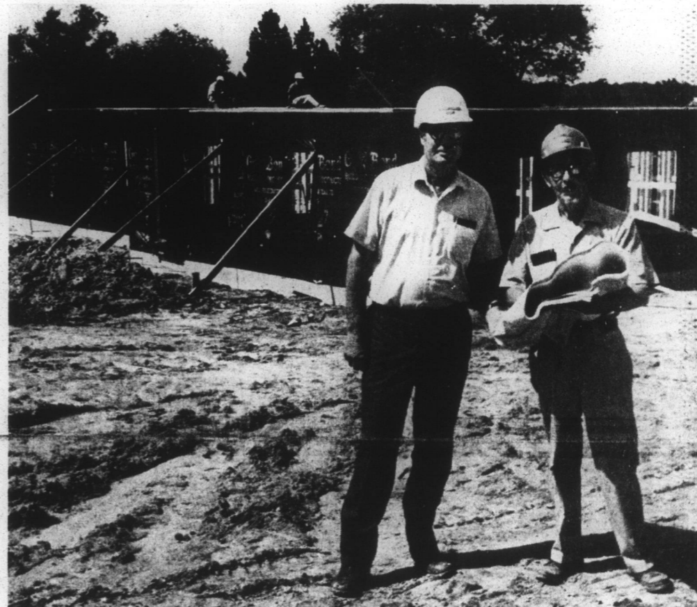
Housing Units Going Up —Work is now progressing on a portion of the 100 units of low-rent public housing being constructed here by Edenton Housing Authority. Ralph E. Parrish, inspector, and Elmer Hobbs, project superintendent for Kirkpatrick & Associates of Greensboro, go over plans at the Twiddy Avenue site where the first units are being built. Sheetz & Bradfield of Atlanta, Ga., designed the project.
