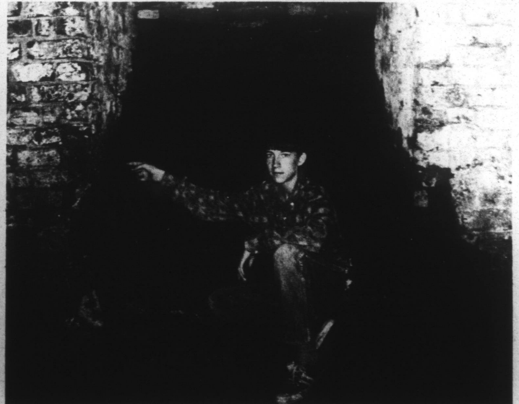
Iredell House Stairway Unearthed—Previously covered by refuse and soil, an outside stairway was recently unearthed in the cellar of the Iredell House. Pictured is David McCall indicating a notch where wooden stairway nosings were inserted to protect the brick steps.
