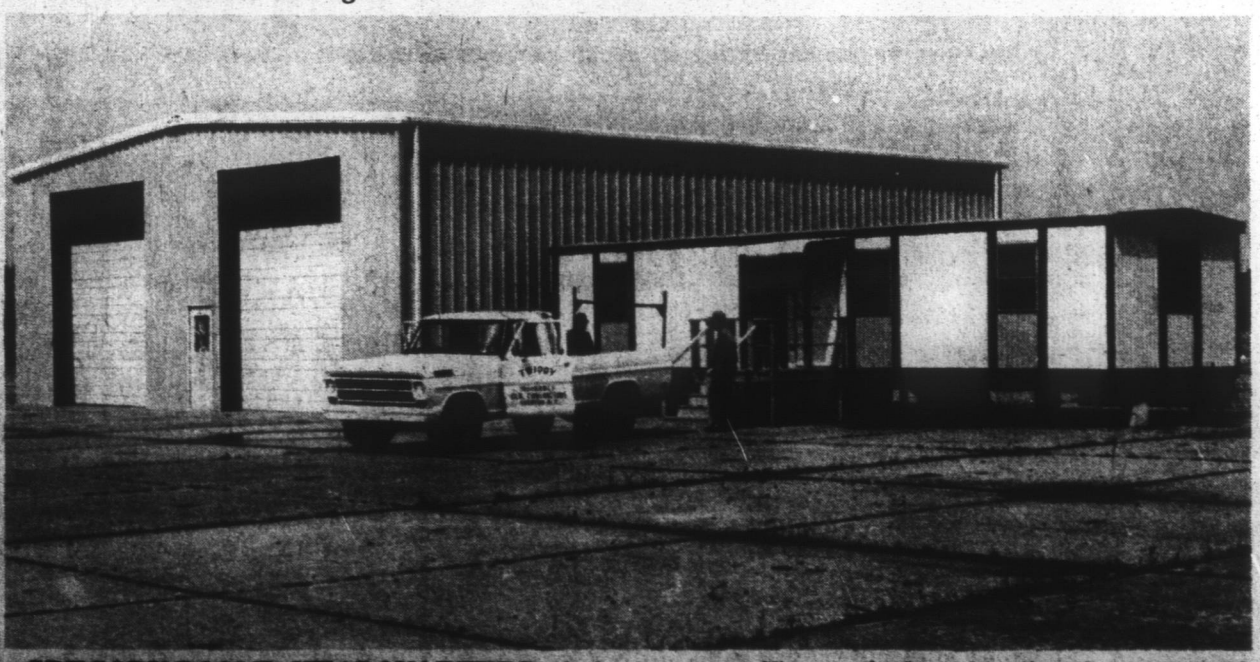
GREGORY-POOLE HEADQUARTERS—A temporary office and shop for the Gregory-Poole operation in the region is being readied at Edenton Municipal Airport. The maintenance operation is expected to employ more than 50 people when it is completed.
