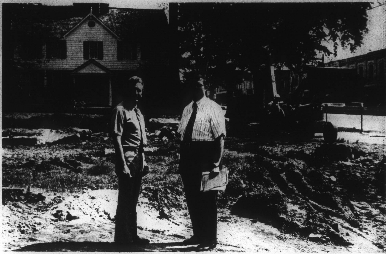
GARDEN WORK BEGINS—Mayor Roy Harrell and town administrator Bill Gardner take a look at initial work that has begun on restoration of the old Cupola House gardens. The town has donated men and equipment to remove the foundation of the old Gooyear building and to prepare the property for fill and grading. It is hoped that most of the restoration of the garden will be completed by October.
