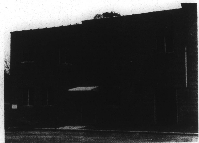
CHURCH DAMAGED —Pictured here is the damaged W. E. Charlton Educational Building of Providence Baptist Church which was heavily damaged by fire early Friday morning. Cause of the fire has not been determined.
