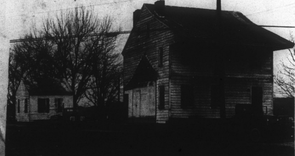
PREPARE FOR MOVING DAY —It is not just an ordinary moving day awaiting out on North Broad Street. It is preparations to move the historic Coke House to the Greenfield section of Chowan County. Worth Hare, moving contractor, has the job of moving the house and surrounding buildings. It is apparent from the size of the house that it isn't a small task.
