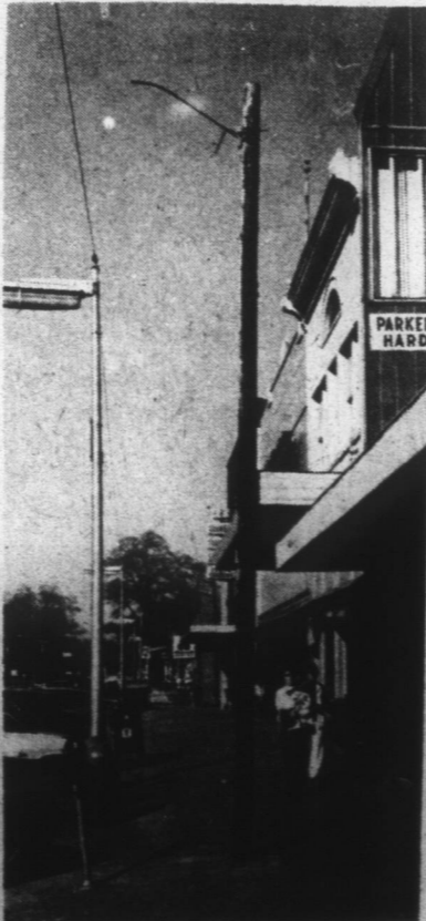
PROJECT BEGINS —The initial legwork of the Downtown Beautification Project has begun with preparing Broad Street for underground electrical conduits. Work began last week on the south end of the street. The pole in the middle of the sidewalk, shown in the right photo, is one of several poles which will provide street lighting while the existing arm-like street lights are removed.
