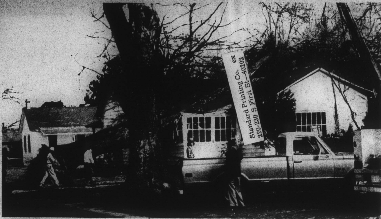
DAMAGED BY STORM —This unoccupied home at Second and Cabarrus streets was heavily damaged Monday afternoon when a twister moved through Edenton and Chowan County. Officials have estimated property damage at $58,000. There were no injuries reported. Other pictures appear on Page 5-A. (Staff Photo by Asbell).
