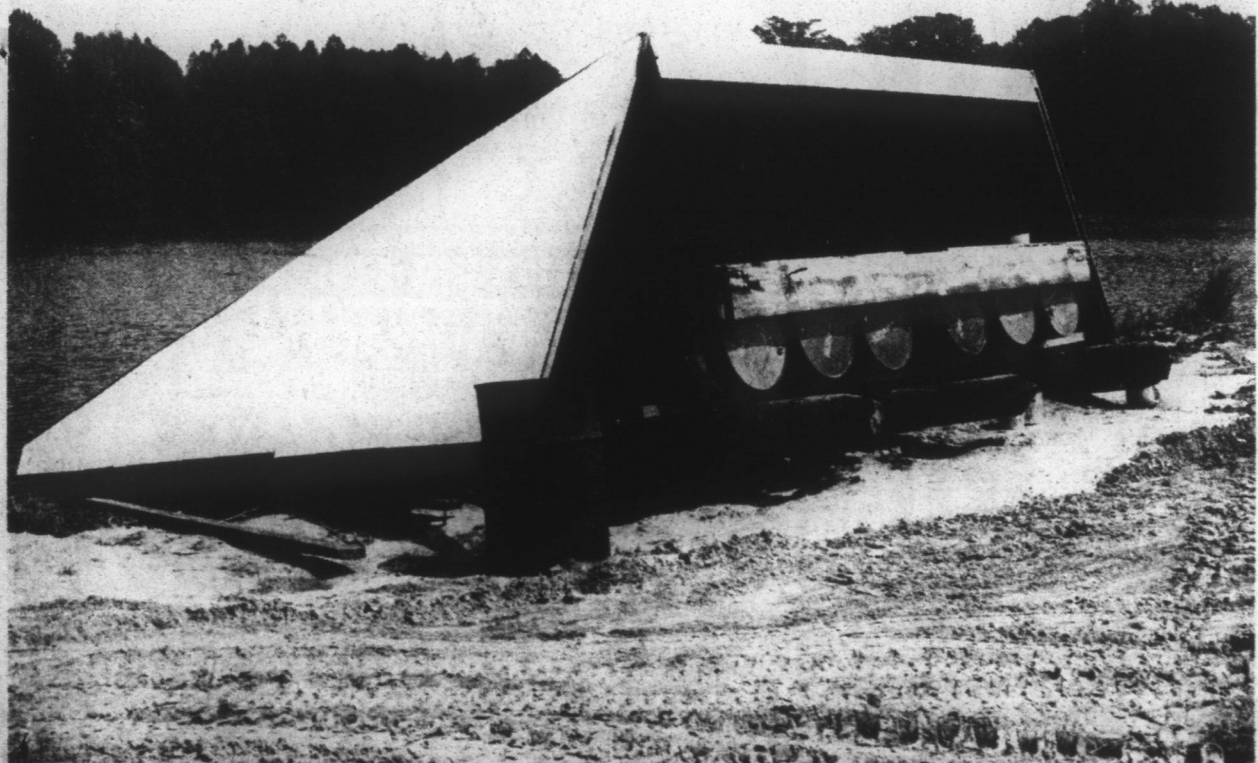
NEW SKI RAMP —Pembroke Water Ski Club has completed construction on a new and improved ski ramp, built at a cost of about $650 by the club members. The ramp features side aprons for safety and a fiberglass surface. It was constructed from treated wood. On May 31 and June 1, the ramp will be put to use when the ski club sponsors a tournament which will include participants from North Carolina, Virginia, Maryland, District of Columbia, and Tennessee. A ski show will be held on July 4 as part of the annual celebration, it was reported.
