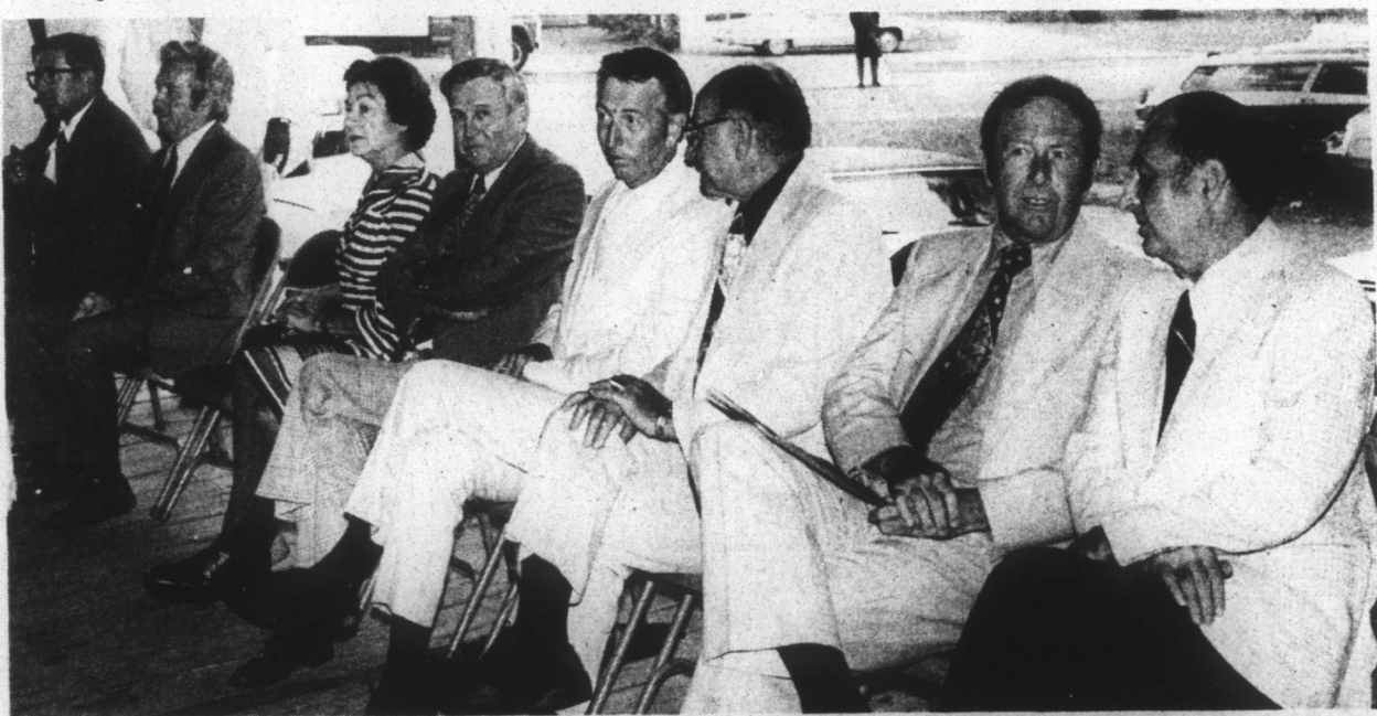
DEDICATION OF WATER SYSTEM — A rainy day in September was the setting of the dedication of the Chowan County Water System, held at the Valhalla Cooperative Exchange. A variety of local, state, and federal officials were on hand to comment on the completion of the $3.8-million project. Shown above from the right is Dr. Bill Turner, NCSU Vice-Chancellor; Paul Parks, state FmHA representative; Rep. Vernon James; Sen. Melvin Daniels; Steve Stevenson of the State Division of Health Services and his wife, Helen; and at far right, Edenton mayor Roy L. Harrell.
