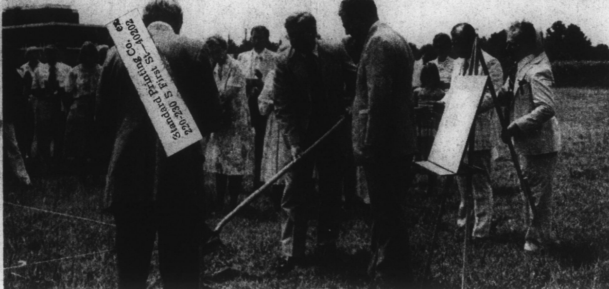
METHODISTS PROJECT BEGINS — Groundbreaking ceremonies for construction fellowship hall-education building for Edenton United Methodist Church was held Sunday marking the beginning of the first of a two phase project. This first phase will consist of a 7,500 foot building to be erected at a cost of $379,000. It will be located on Virginia Road adjacent to Chowan Hospital. The photo above shows L.F. Amburn, Jr., chairman of the Building Fund Committee breaking ground at the new site. Edenton Construction Company was awarded the contract for the project. The second phase will involve construction of a new sanctuary. (See Public Parade.)
