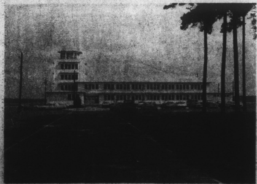
TICKETED FOR DEMOLITION — The tower building, left photo, and hanger at Edenton Municipal Airport have been marked by the Edenton-Chowan Airport Commission for replacement. Both buildings are said to be in such a state of ill repair that it is not economically feasible to launch an im-
