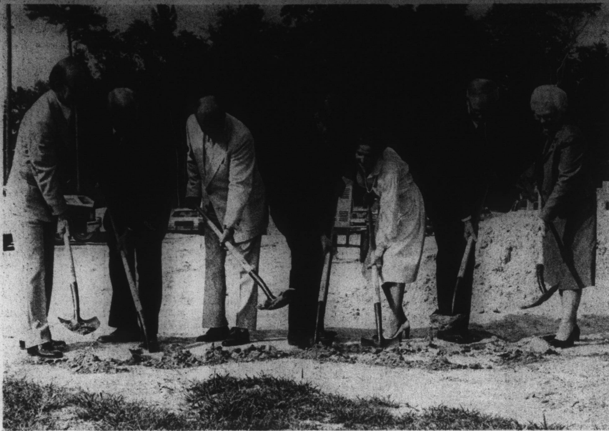
PROJECT UNDERWAY — Groundbreaking ceremonies were held recently at Chowan College for a $2,150,000 gymnasium-physical education center on the campus in Murfreesboro. Playing a key role in the fund raising effort which are continuing is E.L. Hollowell of Edenton, second from left, chairman of "Accomplishing Our Mission." Others taking part in the historic event are, from left: Edgar Parker of Franklin, Va., president of the Chowan Alumni Association; H.D. White of Rocky Mount, chairman, Board of Trustees; Mayor W.W. Hill of Murfreesboro; Mrs. Dorothy Heath Brown, member, Board of Advisors; Chowan President Bruce E. Whitaker; and Mrs. Texie Camp Marks of Boykins, Va., honorary nation chairman, "Accomplishing Our Mission."
