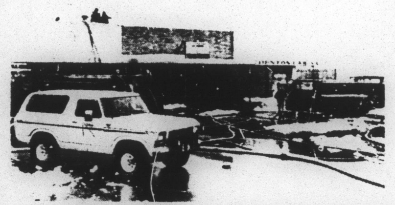
LAUNDROMAT FIRE — A fire between the false ceiling and roof of Edenton Laundromat at Mitchener Village resulted in heavy damages to the facility. Half of the roof was badly damaged as was all of the interior ceiling and wall panelling. Firemen had the blaze under control in about 15 minutes and remained on the scene for three hours afterward. The actual cause of the fire is undetermined pending further investigation.
