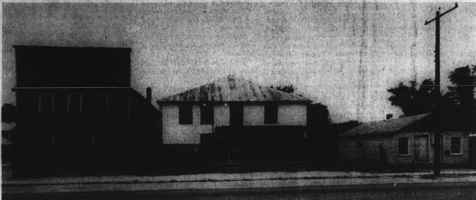
LAST PHOTOGRAPH — This will be one of the last pictures taken of these three buildings located on the 300 block of North Oakum Street. The buildings are included in the five structures
