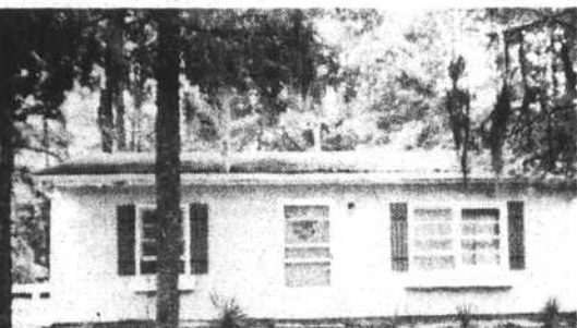
Arrowhead, Canalfront - 2 bedroom, 1 bath, pier, 2 sheds, flue, owner to replace roof.....$27,000.
