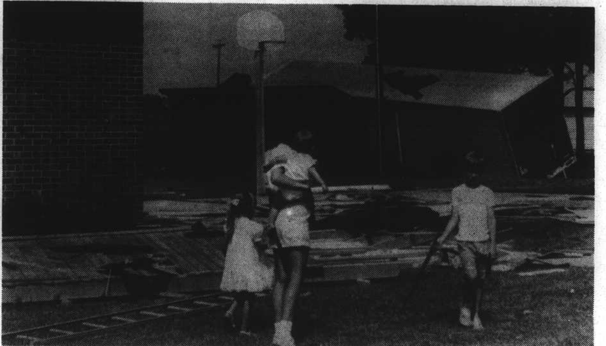
EXPENSIVE SNEEZE —The driver of the tractor-trailer in the background said he sneezed and lost control before the vehicle plowed across a ditch, fence and open field and struck the house and landed to the side and rear of the structure. The truck crossed a driveway where the children of Mr. and Mrs. Jerry Parrish usually play. The family above was one of many friends and neighbors who eyed damage Monday and Tuesday when debris lay strewn about the yard and part of the porch roof could be seen atop the trailer. (Related story and picture on Page 4-A)
